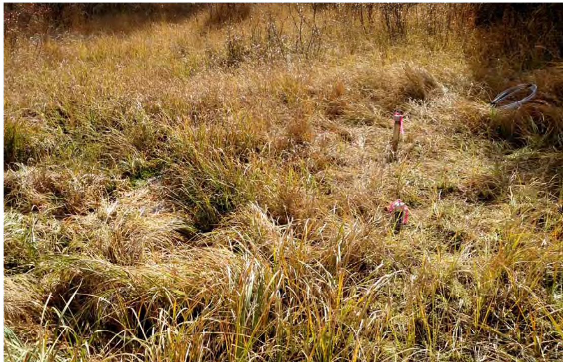
Well FB2 (foreground) and FB1 (background) post installation looking south.
