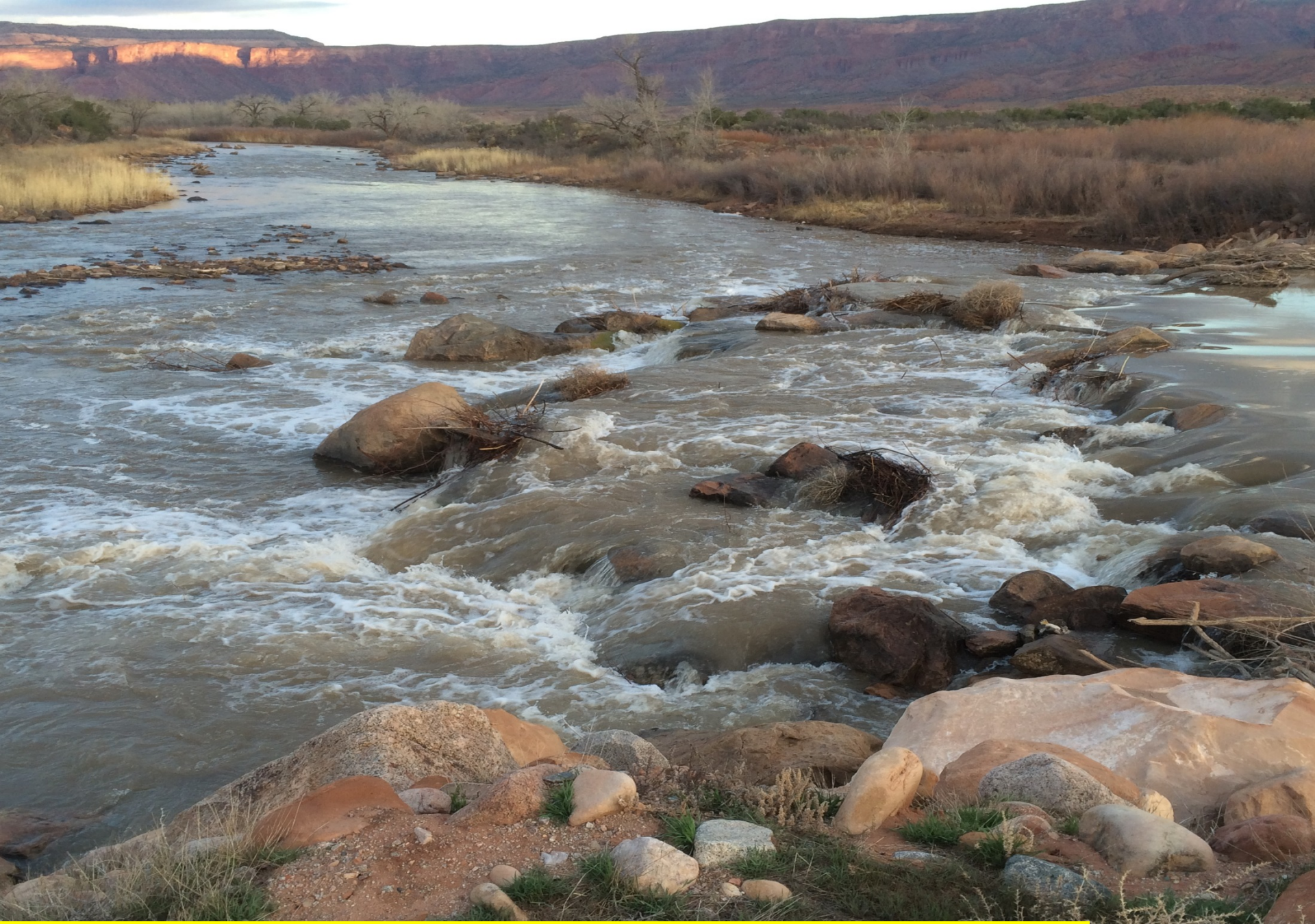
Wines Diversion Structure, semi-permeable, push-up dam
