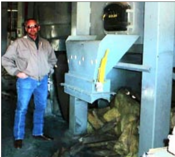
Steve Hall in Eagar is retooling a mill to generate electricity by burning small-diameter wood.
