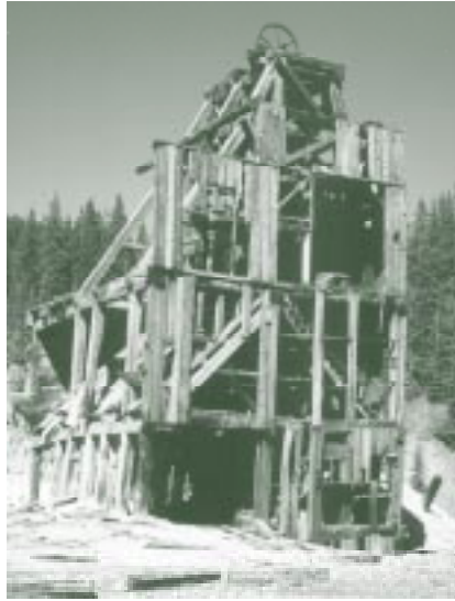
THE SILVER LEDGE HEADFRAME will be stabilized with funding obtained from the Colorado State Historical Fund.
